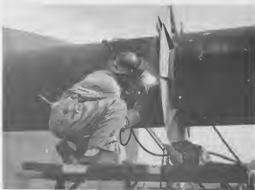
THE SECTIONS were carefully welded together. When completed, the line will be 8,000 feet long, and 3,000 pounds of welding rods will have been used.
